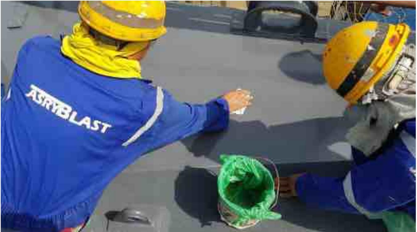
Removing the back film with a pen knife.
