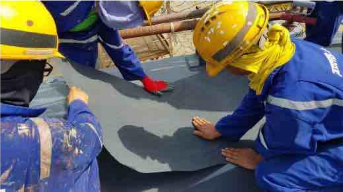
Rolling the Silvagrip panel with a heavy roller. A hand roller can also be used.
